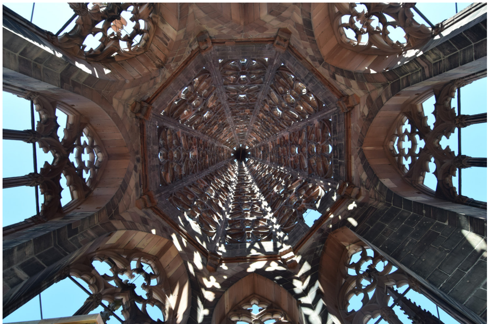
Fig. 2. View from the octagonal hall into the stone pyramid of the Freiburg spire.
