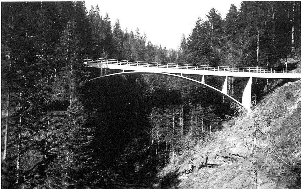
Fig. 23. Maillart's Schwandbach Bridge (1933) – credit: ETH-Bibliothek Zurich, Image Archive/Robert Maillart Archive.
