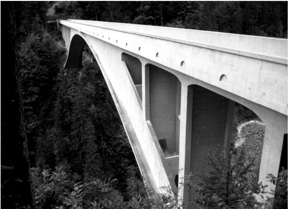
Fig. 10. Salginatobel Bridge (1929) (credit: DZ).
